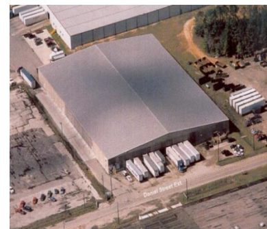
Daniel Street #1 Facility
